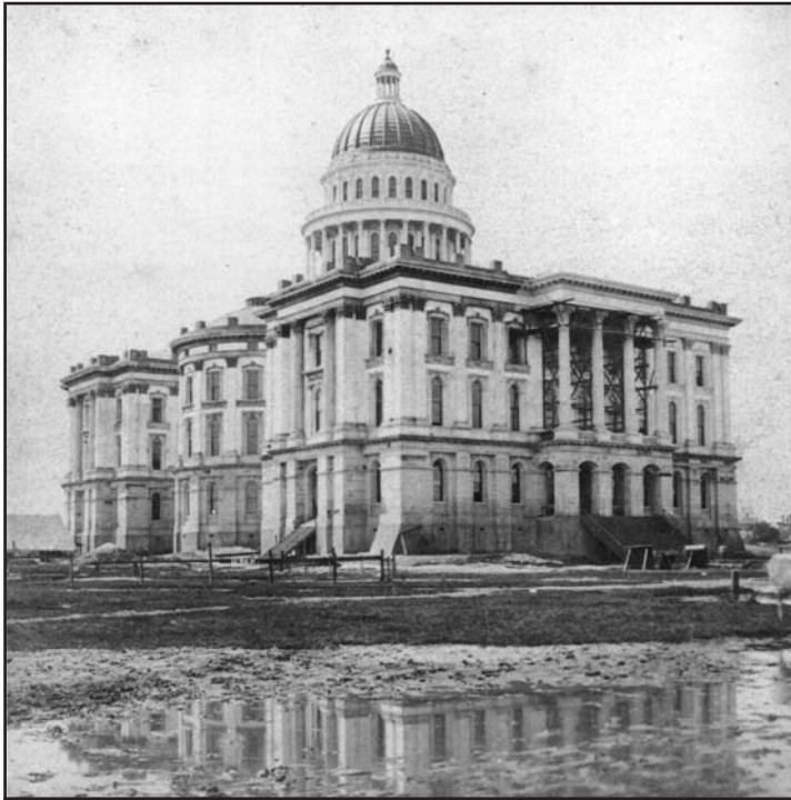
Capitol nearing completion, circa 1872
